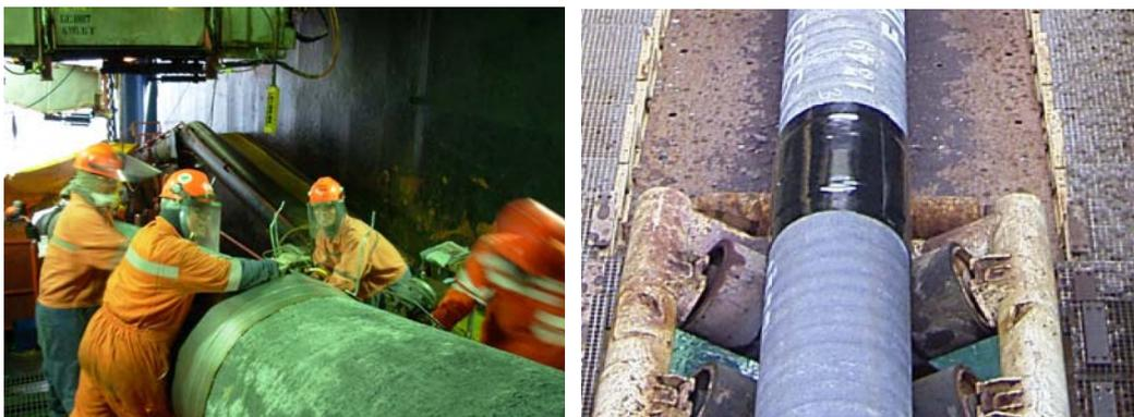
Figure 4.7 Fitting of the infill former in the field joint coating station (left) and a typical field joint after coating (right). The infill former and the concrete coating are approximately flush and aligned.
