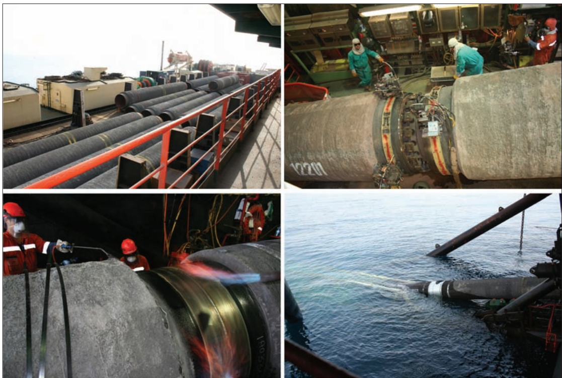
Figure 0.5. Various aspects of pipe-laying activities on pipe-laying barge Castoro Sei. Clockwise from top left: Line pipe on the deck of the Castoro Sei; welding the individual line pipes; preparing the field joint coating over the welded joint; and pipeline entering the water at the back of the lay barge.
