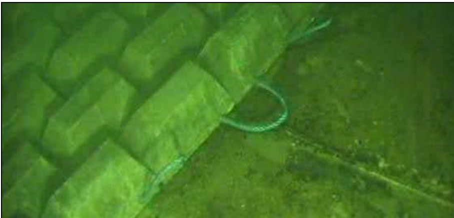
Figure 3.5 LV-S1 cable at the crossing point during the as-built survey.
