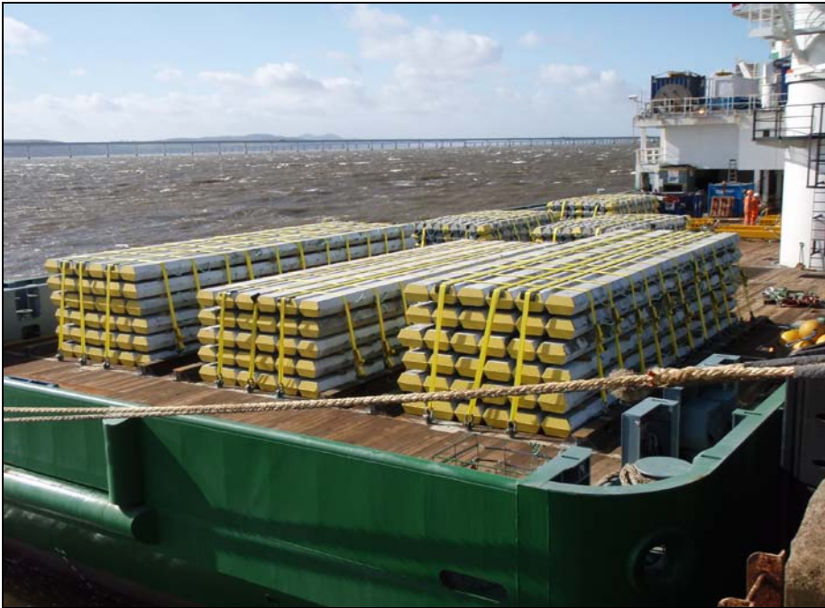
Figure 3.4 Beam mattresses prior to installation in the Swedish EEZ.
