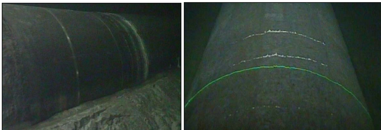
Figure 4.13 Left: Pipeline buckle arrestor observed at KP 513. Right: Minor concrete damage observed at KP 512.
