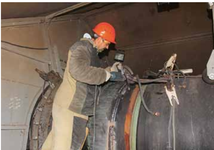
The offshore and onshore segments are welded together in Russia.
