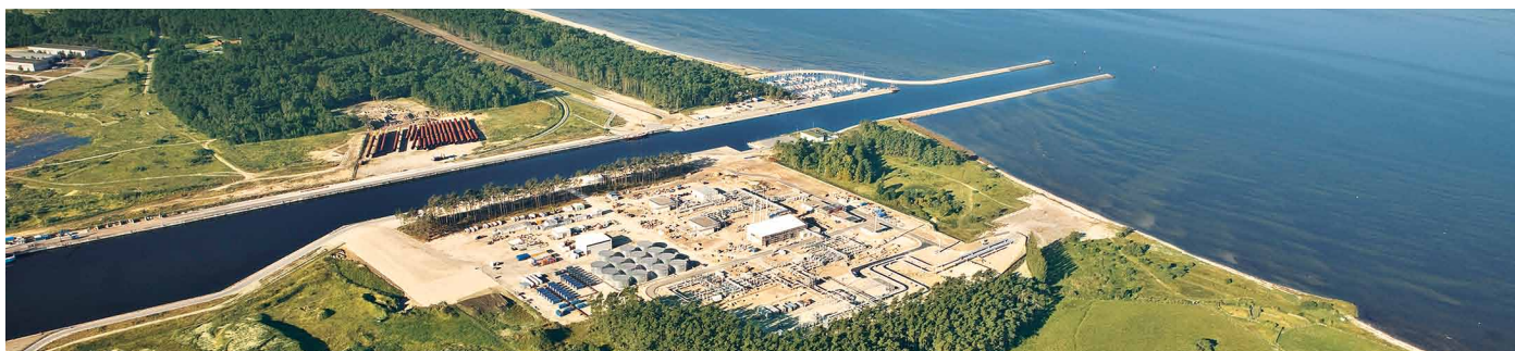
The two lines of the Nord Stream Pipeline system reach land at Lubmin. At the landfall station, the natural gas is purified, measured, and if necessary adjusted to the proper temperature prior to transport.
