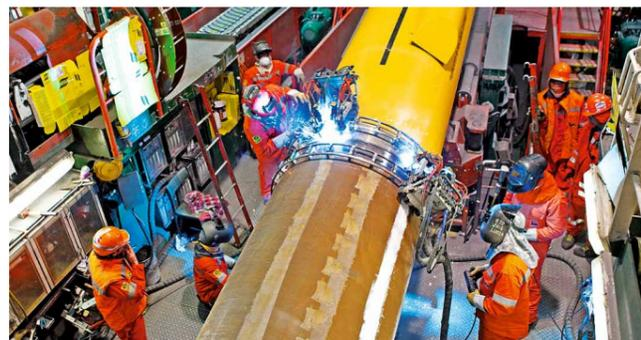
A PIG (Pipeline Inspection Gauge) launcher is welded onto the last pipe of Line 2. The PIGs will later be used to clean and gauge the pipeline sections.
