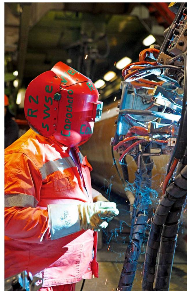
A worker supervises the last welding process. Altogether, some 138,850 welds were performed in order to connect all the pipes laid by the Castoro Sei.
