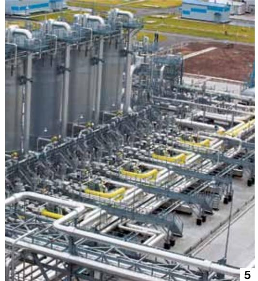
1 and 2) A gas-pumping unit, or compressor, powered by a Rolls Royce motor. 3) The gas treatment facility in the foreground, and the eight compressor units in the background. 4 and 5) The GTU removes condensate from the gas that arrives from the Gryazovets - Vyborg trunkline.
