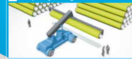
Concrete coated pipes are stored at each of the five marshalling yards located strategically along the route.
