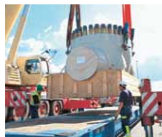
The 102-tonne valve is lifted onto a 26-metre-long lorry with 16 axels.
