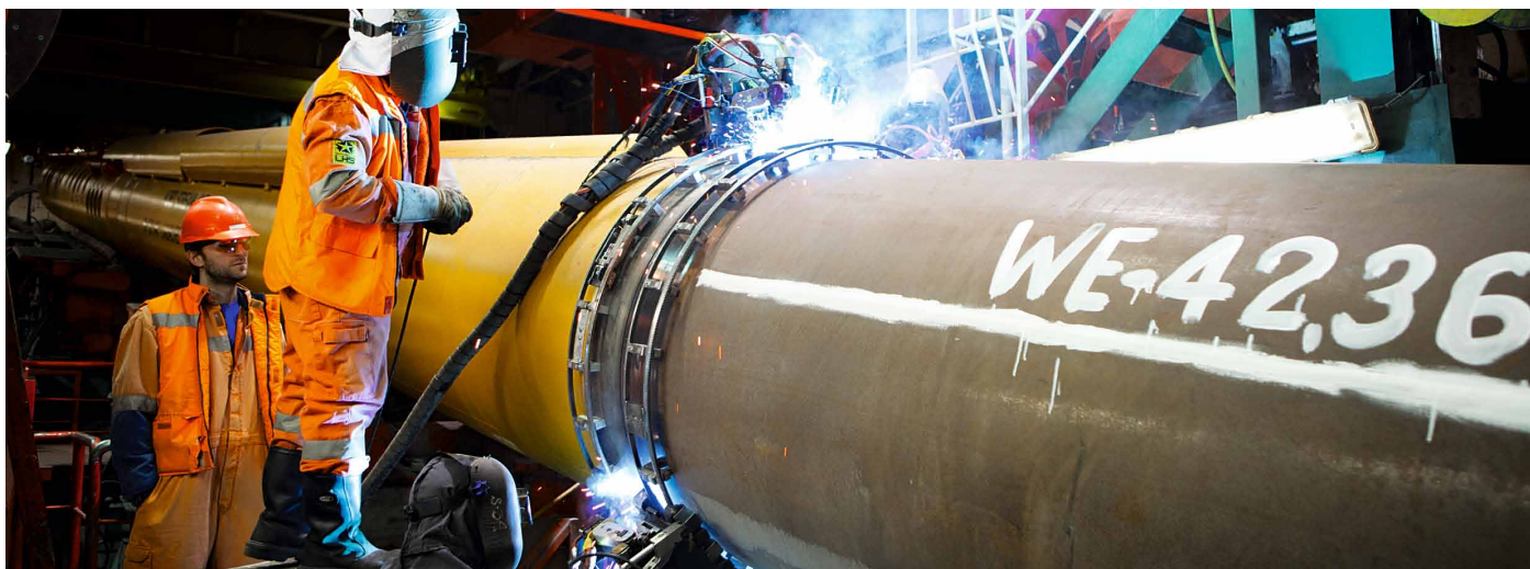
The final pipe of Line 1 of the Nord Stream Pipeline system arrived on the Castoro Sei at the end of April. It was welded onto the third section of the pipeline in May. Line 1 was laid in three sections, which will be welded together underwater this summer.
