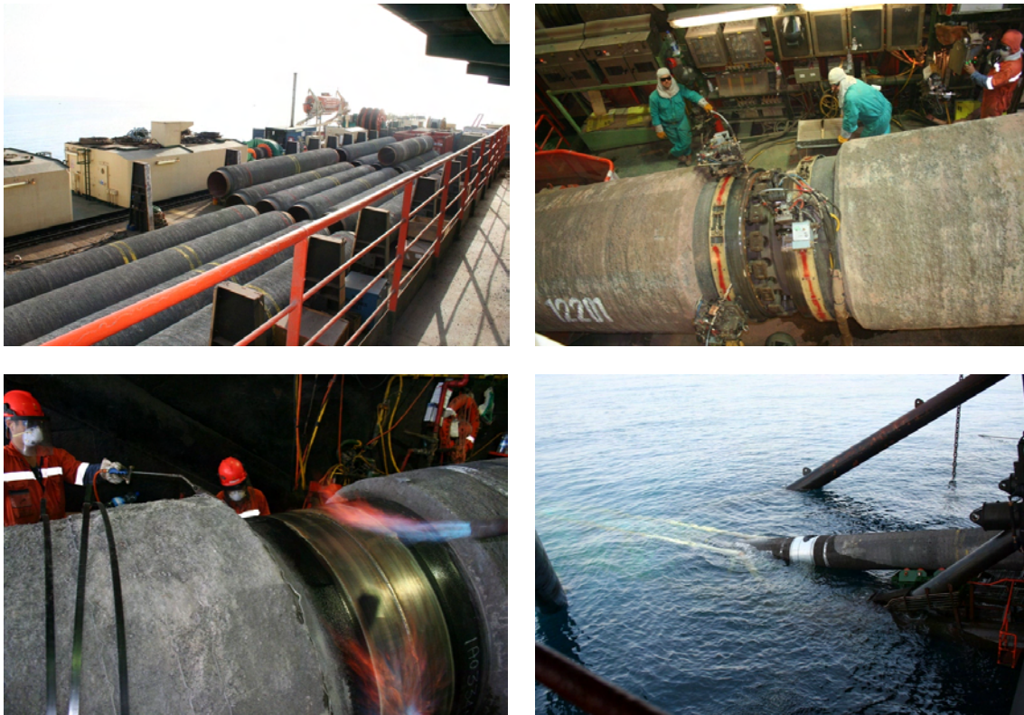
Figure 4.4 Various aspects of pipe-laying activities on pipe-laying barge Castoro Sei . Clockwise from top left: Line pipe on the deck of the Castoro Sei ; welding the individual line pipes; preparing the field joint coating over the welded joint; and pipeline entering the water at the back of the lay barge
